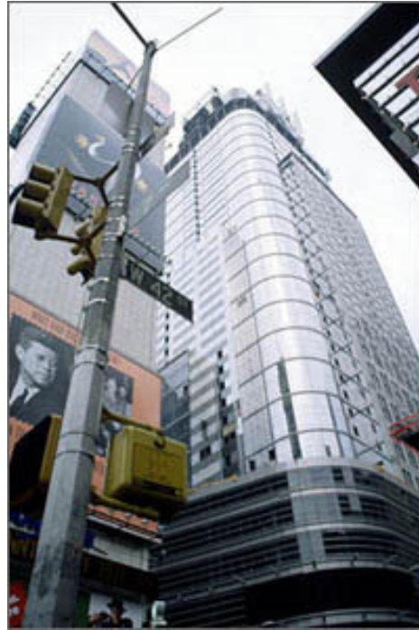
Figure C.15: Thin Film PV Panels Installed in Times Square
